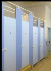
Tin Shui Wai Public Transportation Interchange Public Toilet
